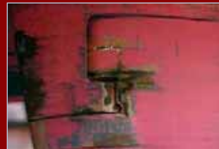
Cavitation damage after sea-trials
